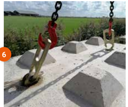
6 Attach the hooks to the anchors and the block is ready to be lifted
