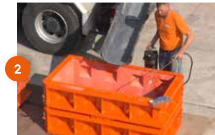
2 Applying oil into the mould
