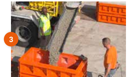
3 Pouring the concrete
