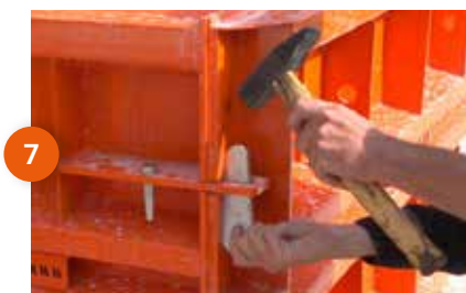
7 Removing pins and wedges
